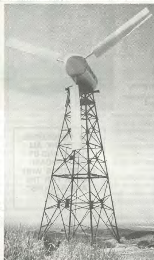
A 200-kW aerogenerator being built at the power station at Carmarthen Bay.
